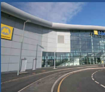
Liverpool South Parkway station with airport link
